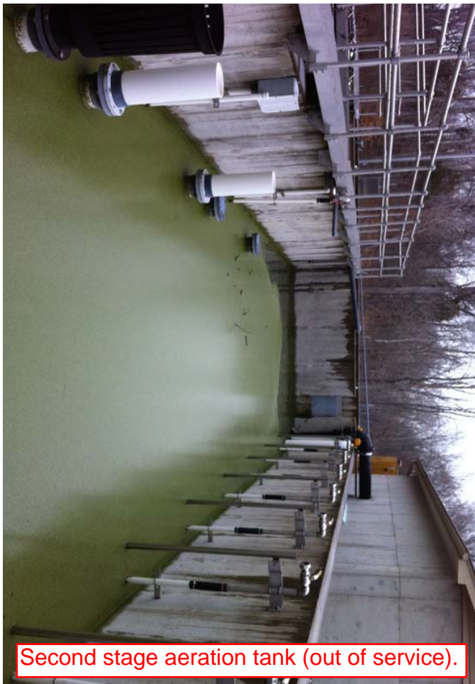
PVC air pipes that have been replaced.
