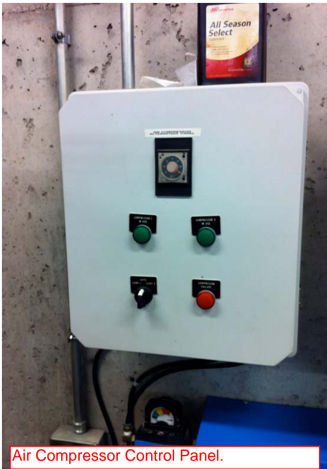
Air compressors for pneumatic controls.
